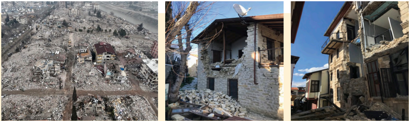
Figure 2 Historical environment damaged in the earthquake 2
